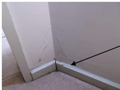
Signature evidence of on-going moisture ingress is clearly visible.
