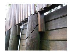
Left – Further securing using stainless steel M12 bolts with 50mm washer plates / suitable coach screws with washer plates. Right – Singular nail fastenings is considered inferior.
