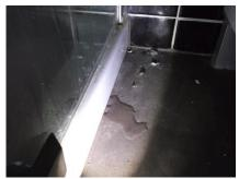
• Employing the services of a trade registered professional to further assess the assumed plumbing leak event and ascertain damage (if any) to local timber framing associated with the bathroom S/W elevation.
